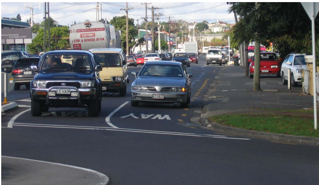
Figure 7.2 View of smaller vehicles approaching the roundabout from Carr Road. Kerb to kerb width is just 5.3 metres.
