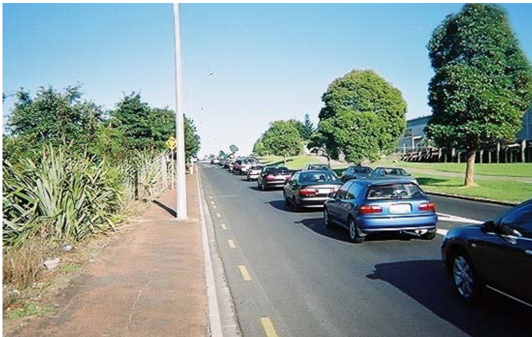
Figure 9.2: Westbound queues on Merton Road during the morning peak. Note the virtually unused left-turn only lane. With a C-Roundabout design, straight-through vehicles can utilise this lane and thereby reduce delays.
